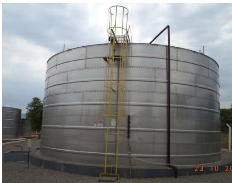
Figura 113. Reator UASB
