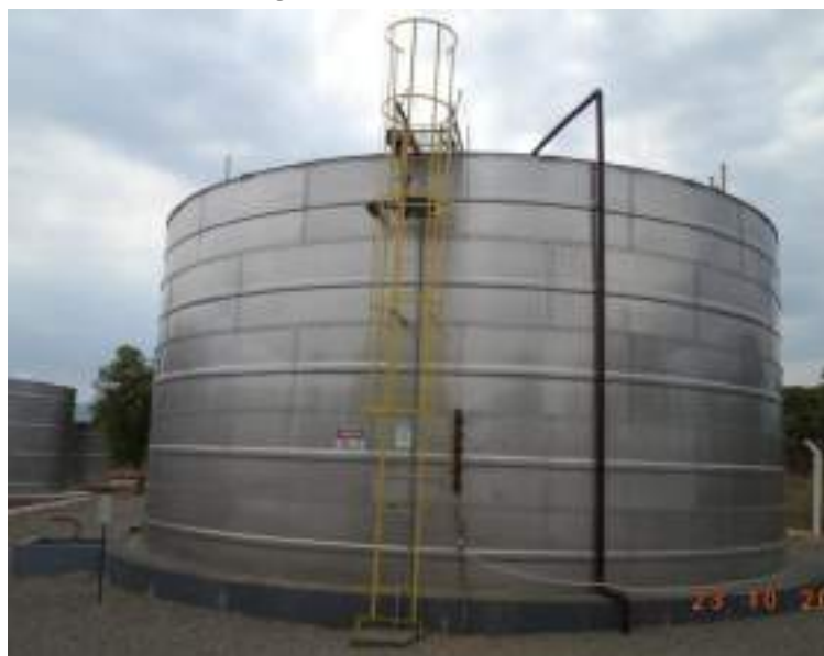
Figura 113. Reator UASB
